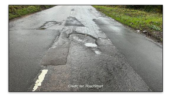
A familiar sight along many roads, some deep enough to cause serious tyre and wheel damage. One of the problems is that repairs get carried out to fill in the potholes but with rain and frost they reappear in a short space of time and the repairs have to be repaired.
